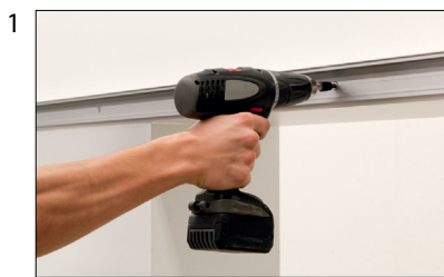
Fixing the track profile from the front
