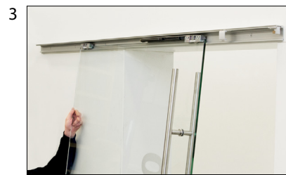
Mounting the door leaf in the track from the front
