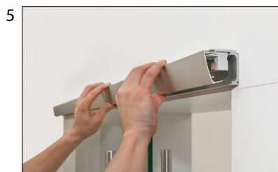
Clipping the covering profile into position
